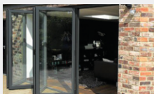
Bi-fold doors Ultrarroof's beam is strong enough to allow for bi-fold or sliding doors up to 4m wide without any extra support
